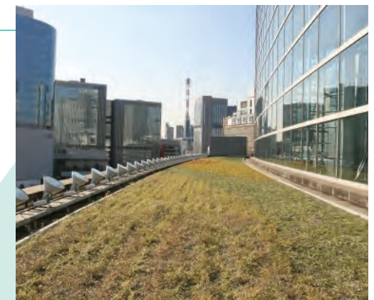
Roof of a conference room in the Glass Building
